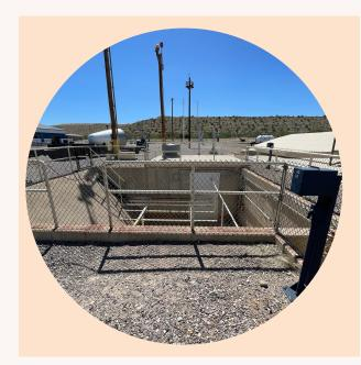
Between the silo door and the pole with the Thunderbolt siren you can see **two pits**. One is enclosed with a metal cover, while the other is open and surrounded by a handrail. The covered pit contained an **electric power transformer**. It was used to supply the complex with **480-volt** electricity and it was connected to a distribution center at Level 3. At Level 3, there was an emergency generator used to supply electricity to the complex in case of a blackout.
