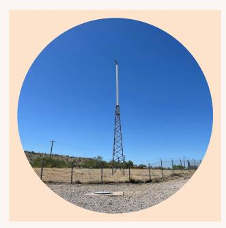
Close to and outside the fence, on the right of the main access portal, you can see two other examples of soft and hard (pole-like) antennas. The one on the left, with the square base, is the soft **IRCS Antenna**. This antenna was designed for frequency diversity. This means that it could operate on many different frequencies at the same time. This antenna would deliver the order to launch, as it would be a direct link to Strategic Air Command (SAC) Headquarters.
