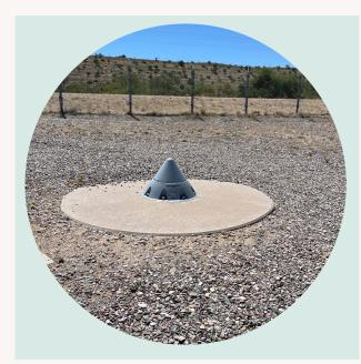
A semi-hardened, cone-shaped **Ultra High Frequency (UHF) Antenna** was used to communicate with helicopters and other aircraft. These aircraft would be linked to the Command Post and Strategic Air Command. The latter would be an airborne command post known as "Looking Glass," and commonly referred to as the "Doomsday Plane." This aircraft would give the orders to launch the missile.
