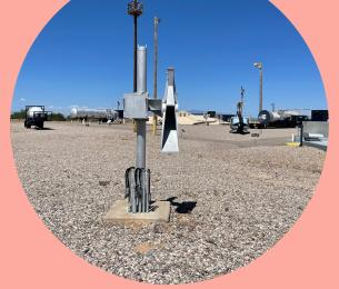
**surveillance security system**. Pairs of TPS (tipsie) units are located at each corner of the silo (short scoop poles) and also on each side of the Launch Control Center air intake shaft. These shorter poles on both sides of the air shaft would project a beam that would be triggered by motion. The TPS-39 sensors had their own battery backup; in case of total power failure they could stay on for a couple of hours.
