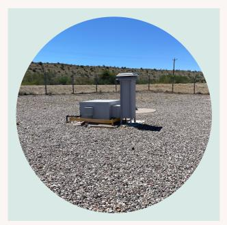
There were three **air shafts** that provided air circulation to the underground complex. Two were for fresh air intake, while one was for air exhaust. The shafts were made of corrugated metal pipe sections 3 feet (1 m) in diameter that opened to the surface; two are next to the silo door. One air intake shaft was built next to the Launch Control Center and provided the crew with fresh air. It was also used as an emergency exit. Now an AC unit sits on top of the hole.
