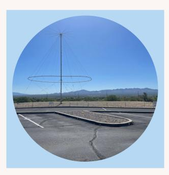
The biggest antenna used for communications was the **High Frequency Short Antenna**, or discage antenna. It is viewable in the parking lot of the Museum and resembles a Christmas tree. This antenna was "soft," meaning that it would not survive a nuclear blast. It is operational to this day.
