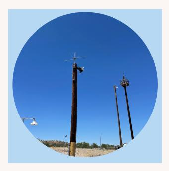
The **Radio-Type Maintenance Network (RTMN) Antenna** can also be seen. It sits atop a pole close to the access portal. This pole is also equipped with the **Voice Signaling System (VSS)** speaker. This antenna had a more localized use, as it would allow communications between the crew and the maintenance teams working topside. The antenna could be disabled when not in use. The **VSS** would be used to make public announcements from the Launch Control Center to the topside crew.
